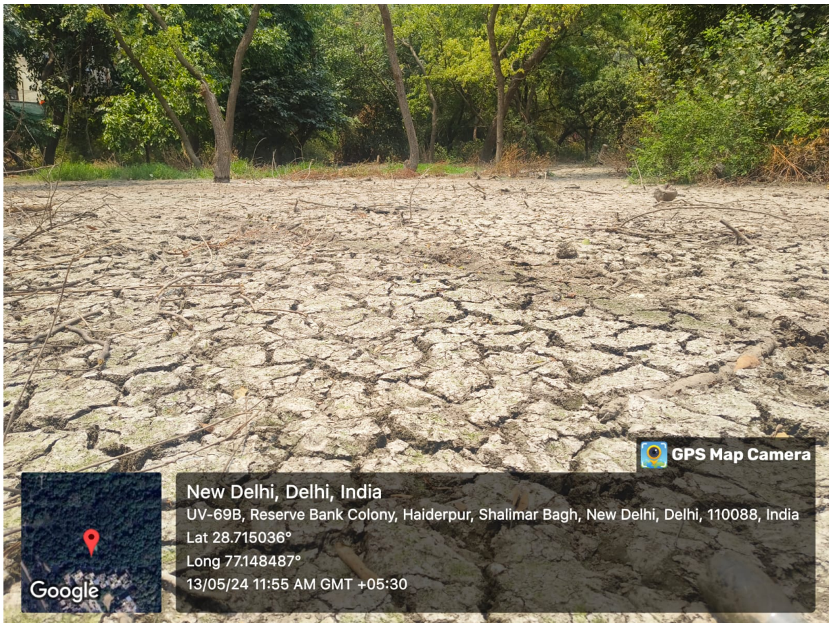
Before/After of the picture of the site
